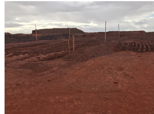
Iron Baron bioremediation pad
